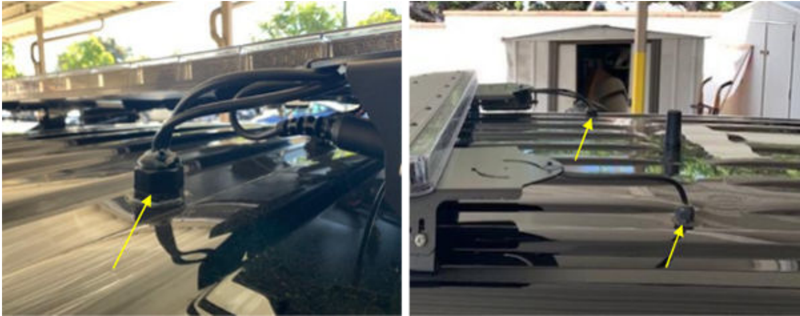
Figure 16: Routing Cables Through Roof Holes
