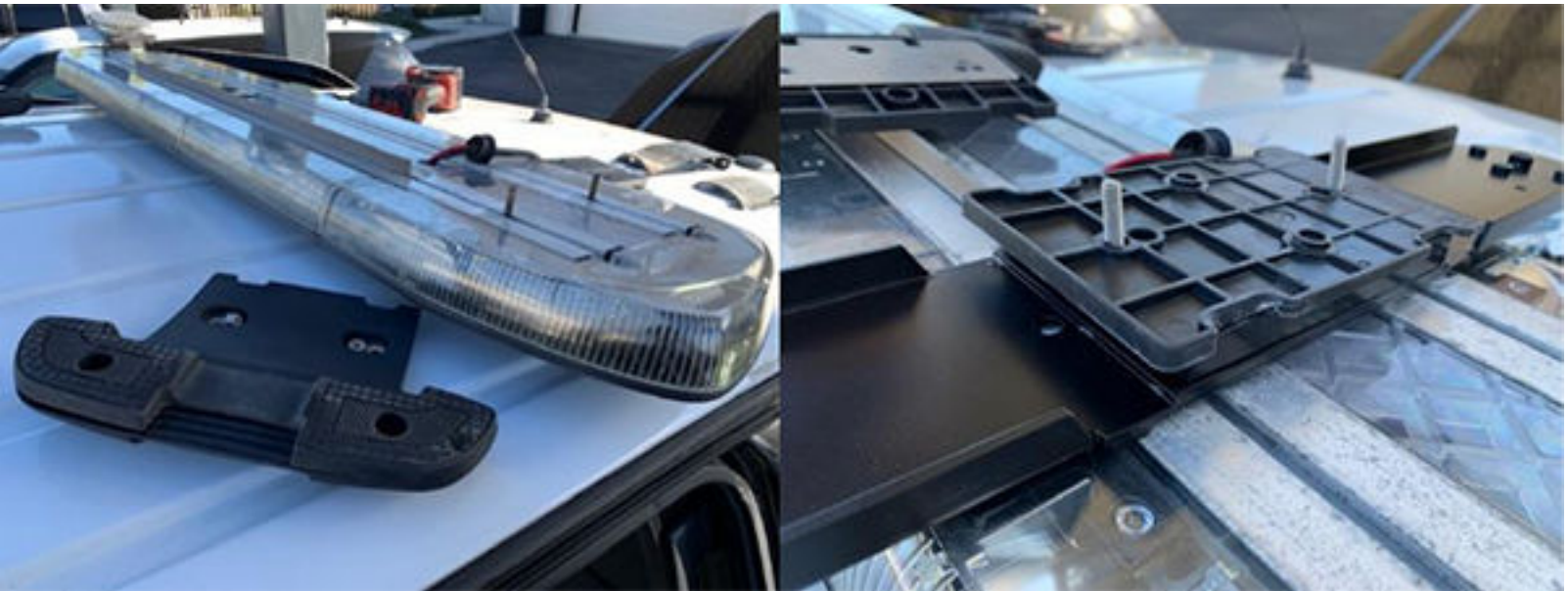
Figure 29: SoundOff Install Process
